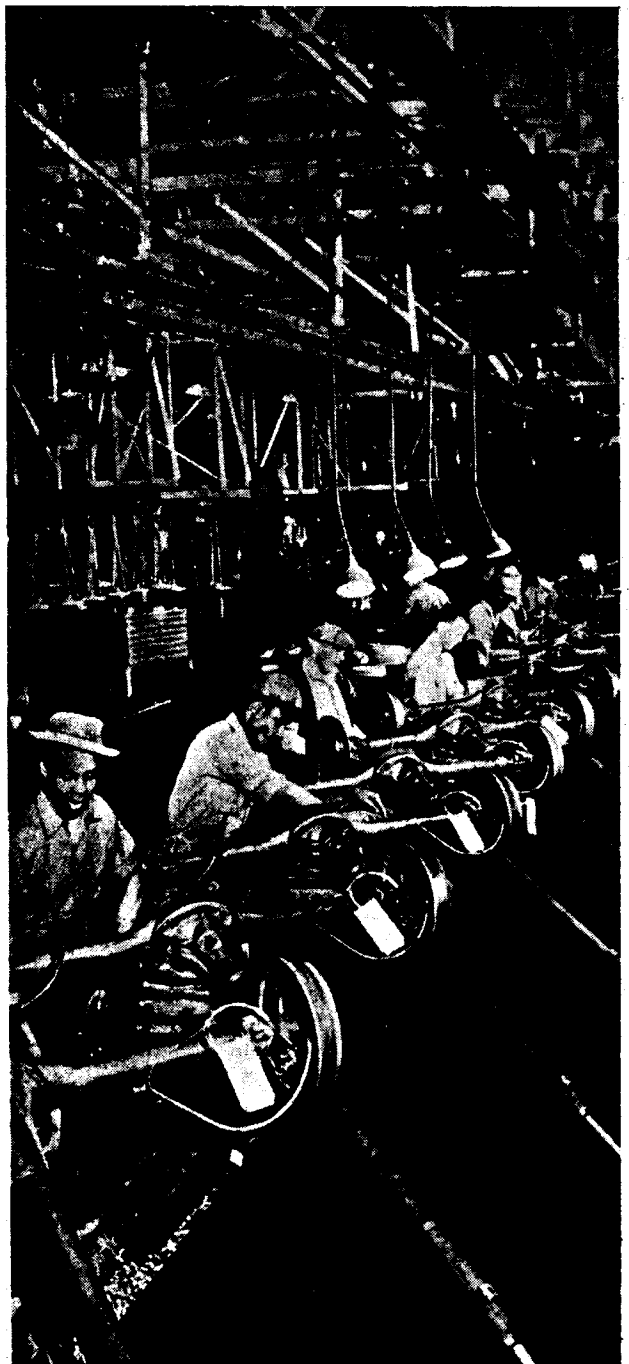
Workers on an auto plant assembly line. Photo from NY Public Library Picture Collection/Liberation
